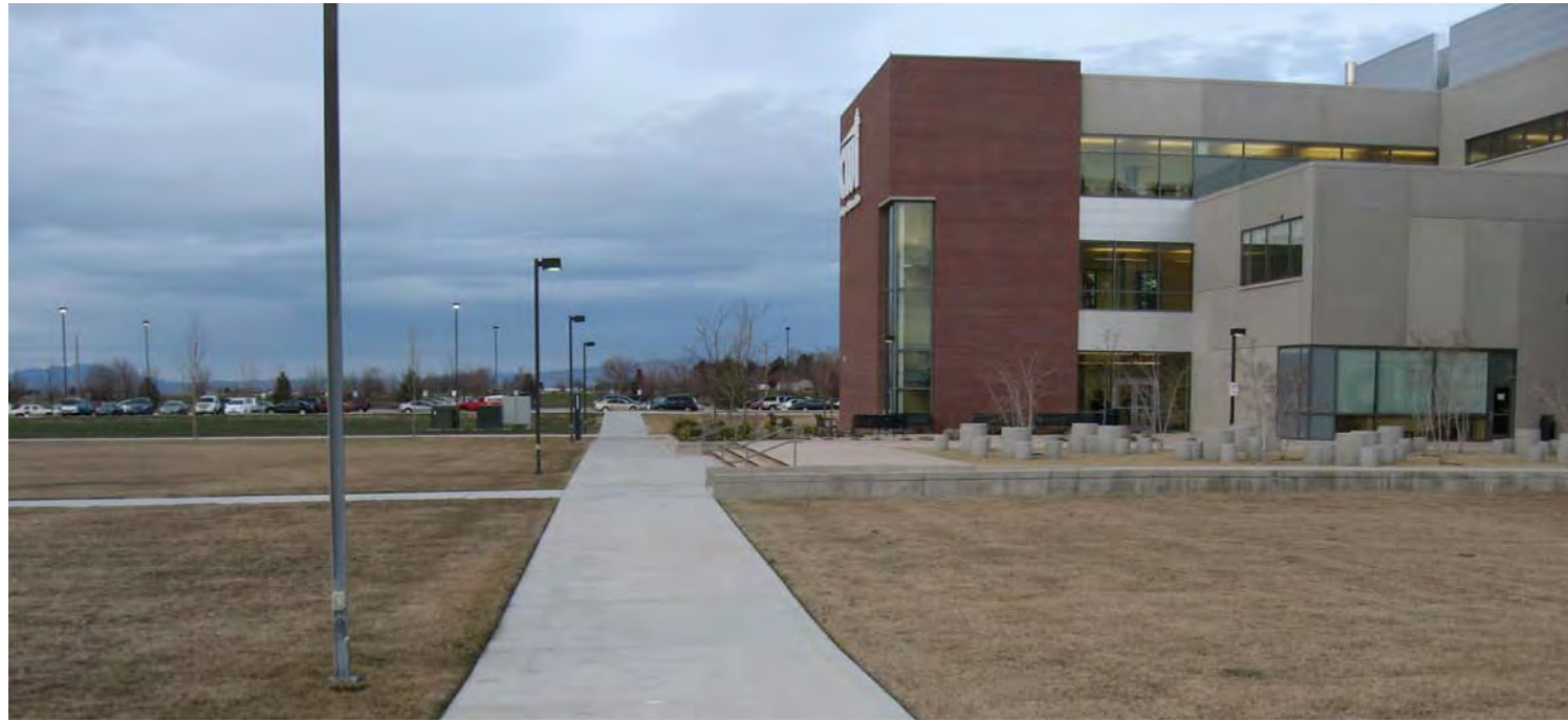
CWI building courtyard and pathway.
