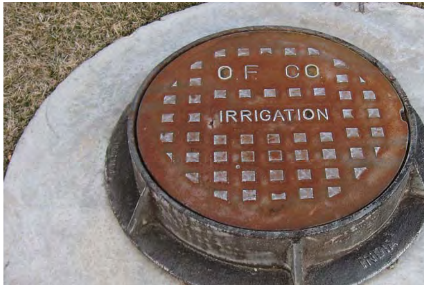
Campus utility access.
