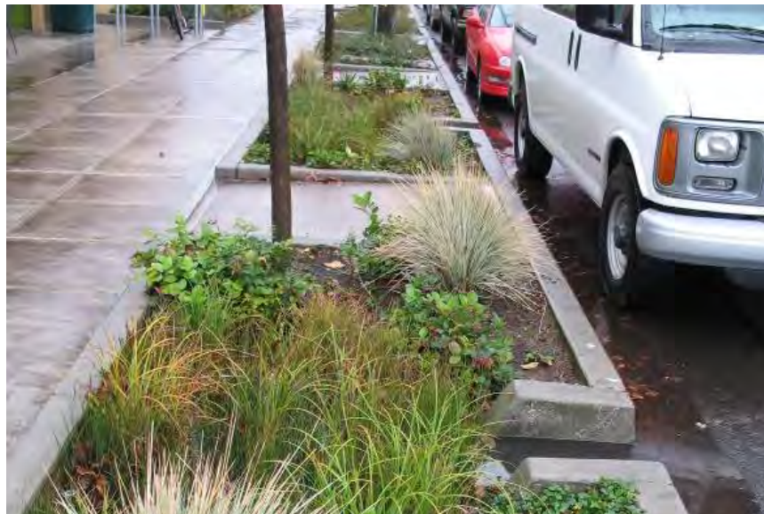
Storm water swale.
